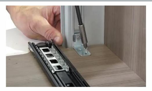
Screw -L connector on the carcase
